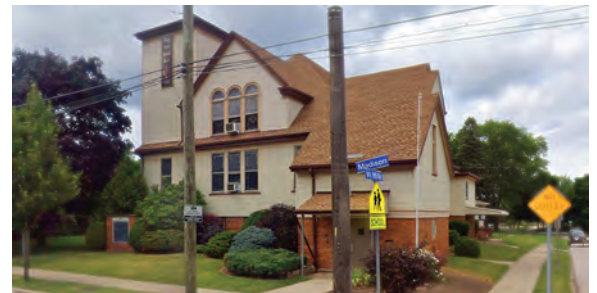
Improvements and renovations to RRUMC's Cleveland Campus.
